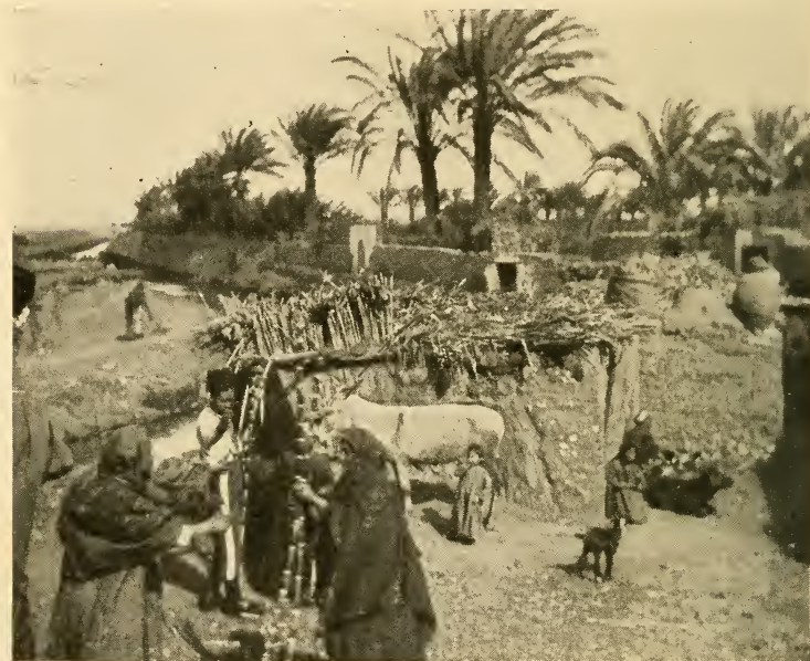
The Egyptian fellah dwells in a hut of reeds and mud
